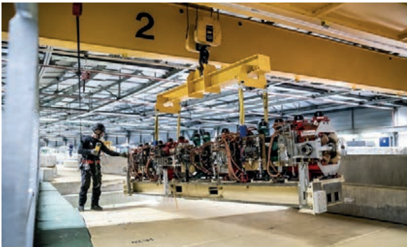
Fig. 1: Dismantling of the third-generation source began in December 2018. By March, nearly 1800 tonnes of material had been removed from the storage ring tunnel.
